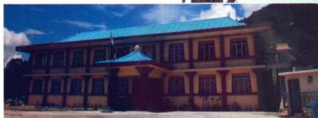
Fig. 1 : Laboratory and administrative Building of the institute
